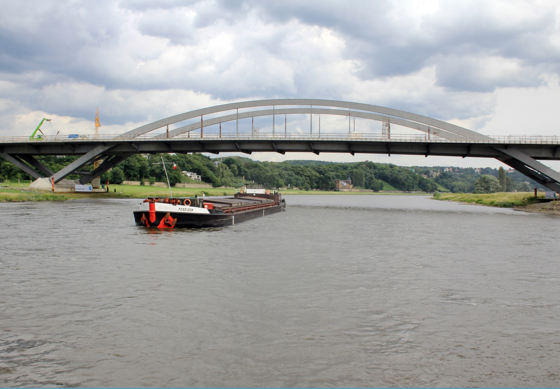
Waldschlösschen Bridge, River Elbe, Dresden, Germany
