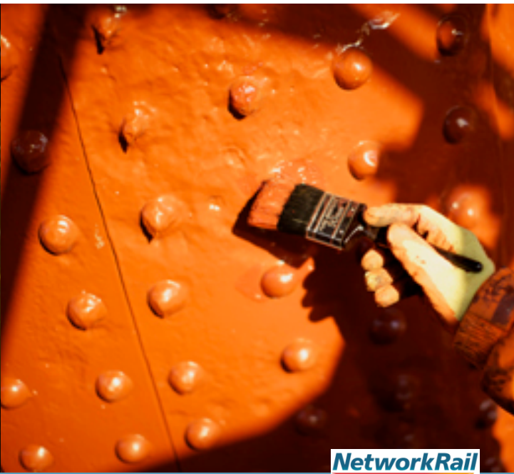
The new paint system requires the application of three layers of paint (images: Duncan Sooman)
