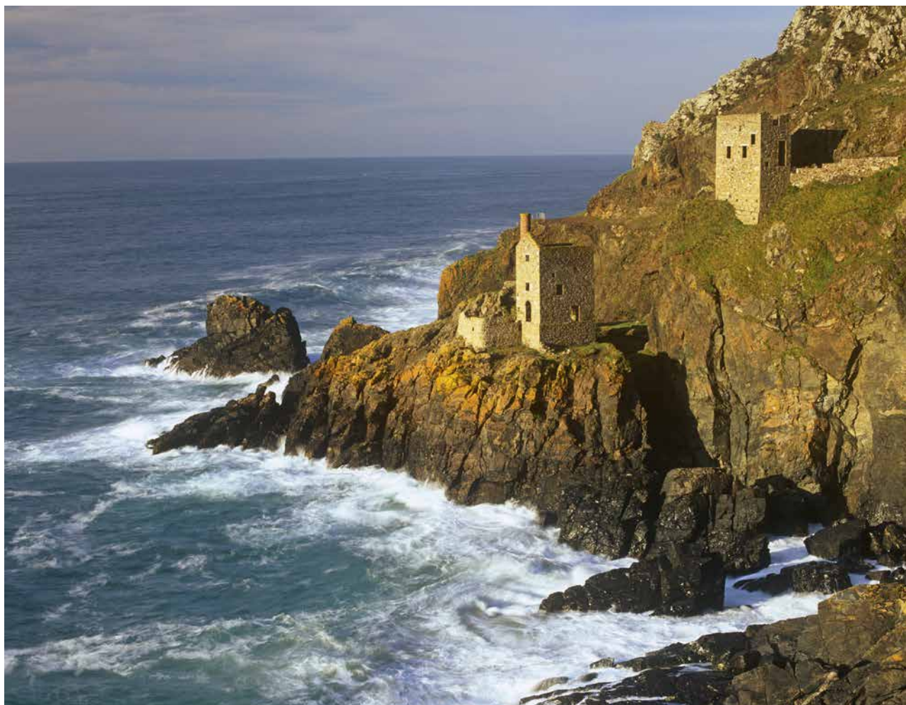
The abandoned beam engine houses of the Crowns section of Botallack Mine near St Just, Cornwall. The steam-driven engines were used for pumping water, and conveying ore and miners up and down, when the St Just area was an important centre for mining tin, copper and other minerals © NT Images/David Sellman
