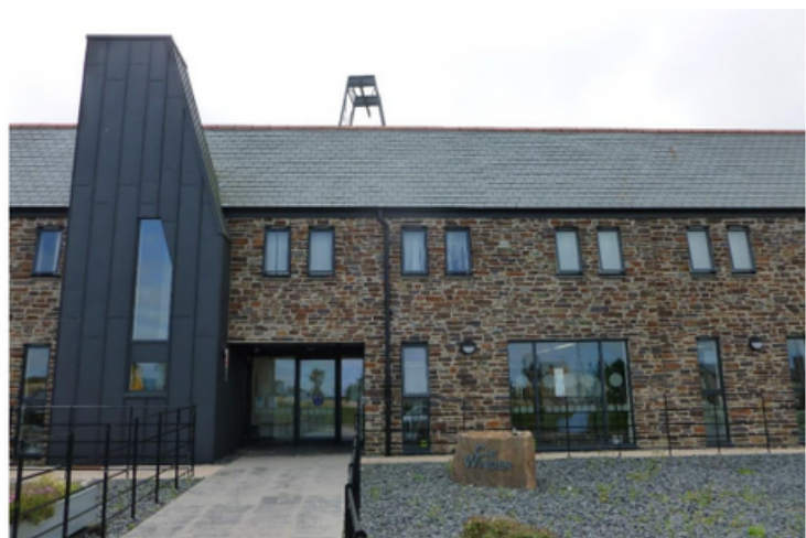
Chy Winder received the WHS Best New Building award for the way in which the building blends into the surrounding mining landscape.
